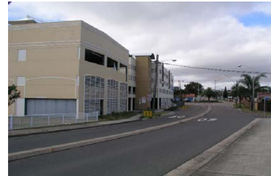
WILFRED BARRET DRIVE (LOOKING SOUTH EAST)
